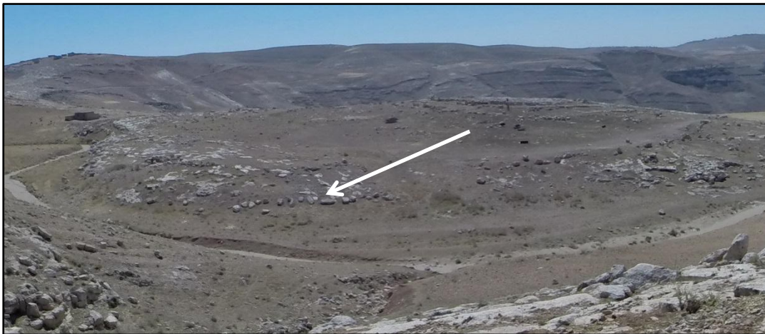
Figure 4 Large stones fallen down from the outside wall at the western side of the central site (arrow).
